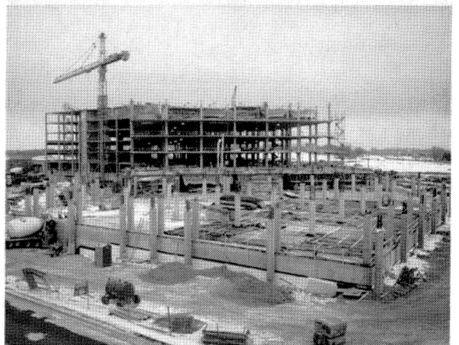
FIGURE 1.22 Construction of a Corporate Office Facility
